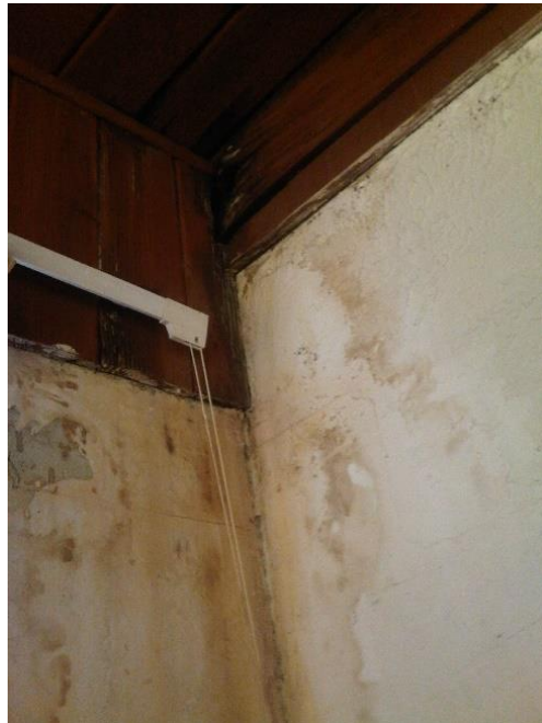
Roof leak trickled down the wall
