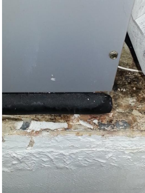
A/C Wall unit drain got clogged
