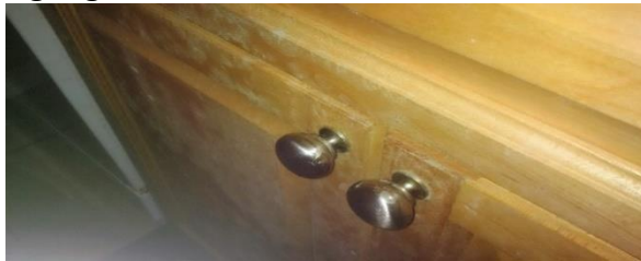
Light green mold dust on cabinet door
