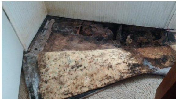
“Mother nature takes back what is hers.” Mold is rotting these plywood and beams under this carpet in a mobile home.
