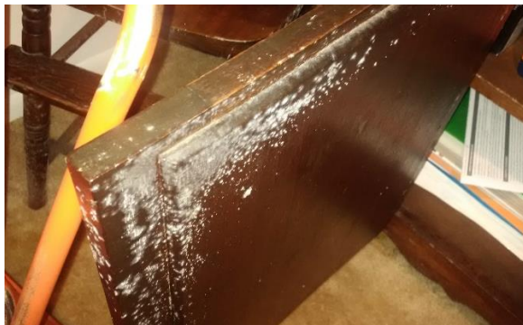
White mold inside the cabinet
