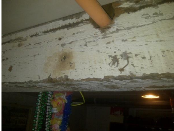
Mold is eating away at this beam
