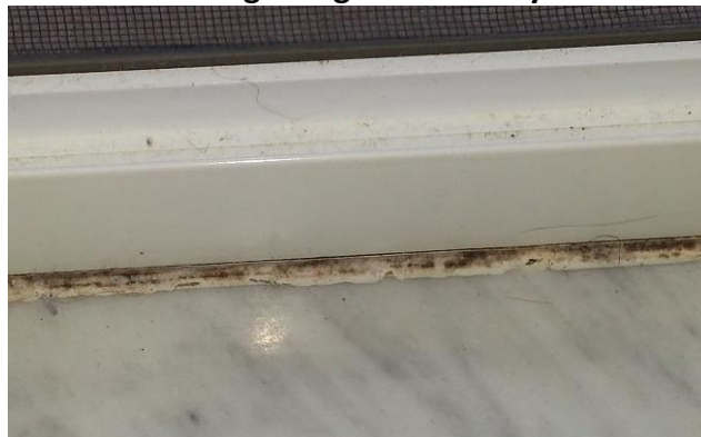
Grout & Caulking being devoured by mold
