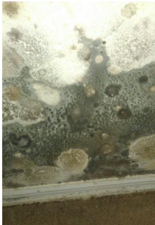
Blue mold behind a kitchen cabinet with the sink
