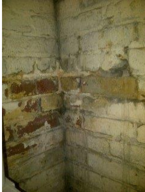
Gold mold on a brick wall painted white.
