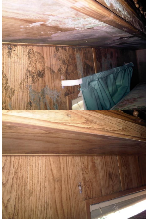
Roof leak trickled down the wall
