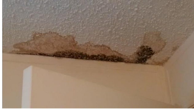
This ceiling leak created a big fuzzy ball of black mold
