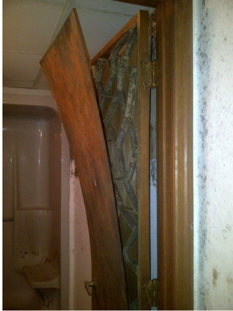
Door separating full of olive green mold
