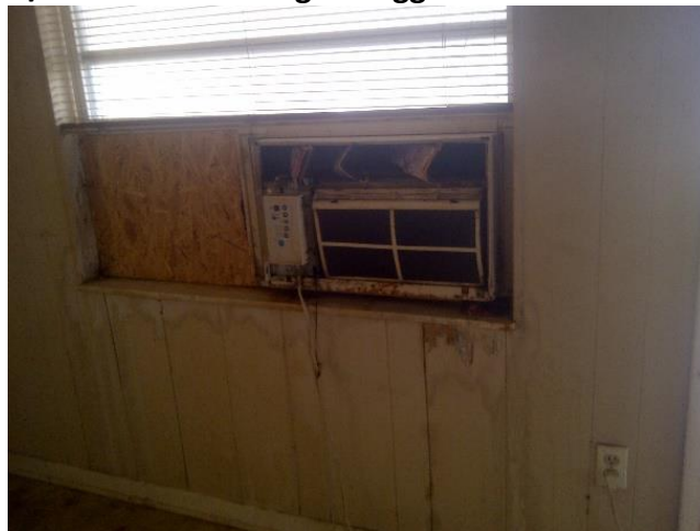
A/C Wall unit drain got clogged
