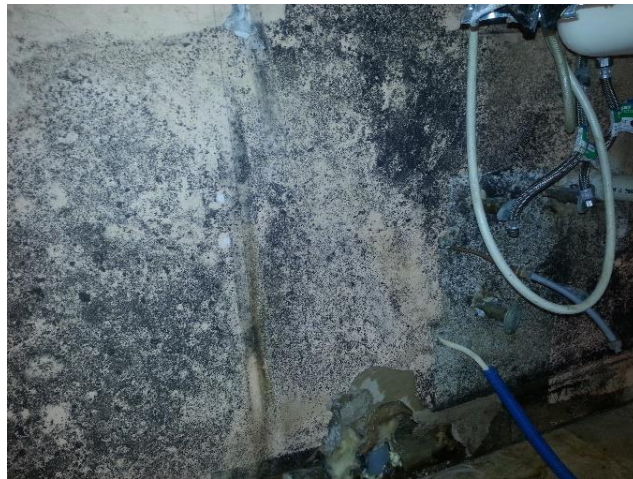
Blue mold behind a kitchen cabinet with the sink
