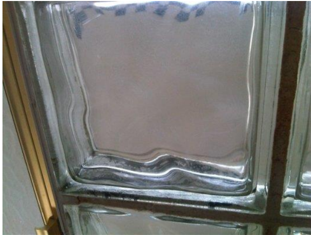
This glass wall had mold growing inside the glass blocks.
