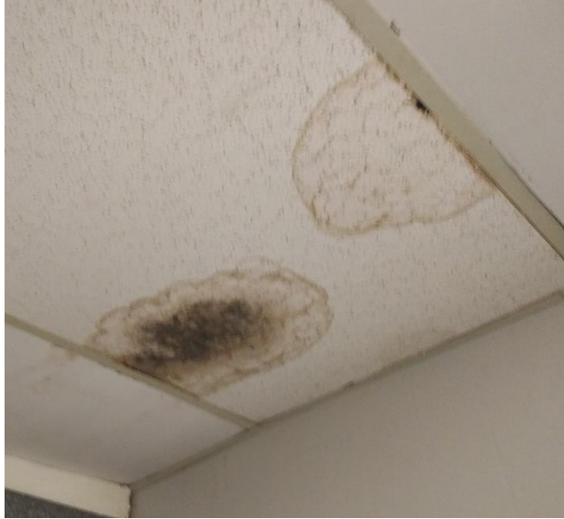
A roof leak created a spot on the ceiling and warped paneling
