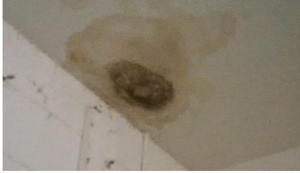
Mold is eating away at this beam
