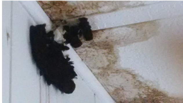
This ceiling leak created a big fuzzy ball of black mold
