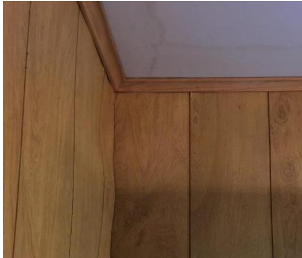
A roof leak created a spot on the ceiling and warped paneling
