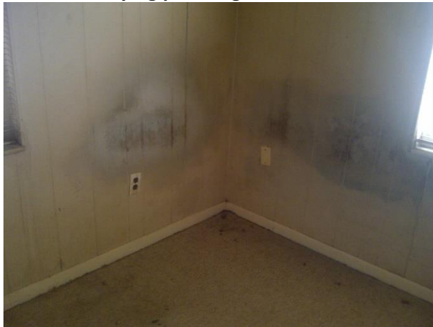
Mold is decaying paneling
