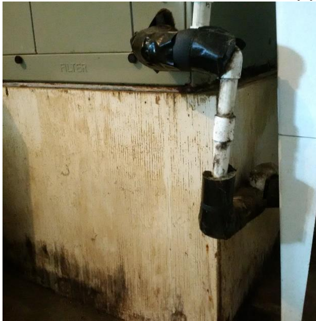
A water leak in an A/C ran down the wall & pipes
