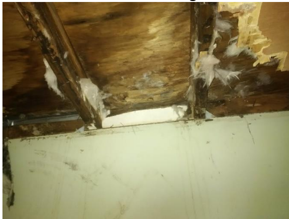
A roof leak can start in one area, travel down rafters (2x4's) and show up inside the home on different parts of the ceiling or on walls. Black and white mold growth seen here.
