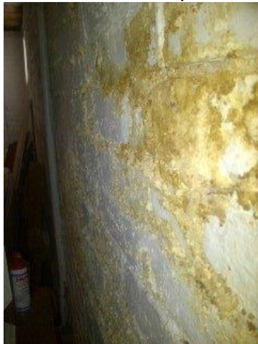
Gold mold on a brick wall painted white.
