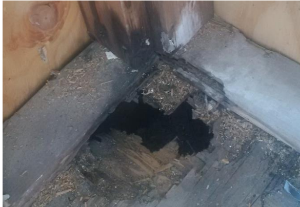
Mold ate a hole through the floor
