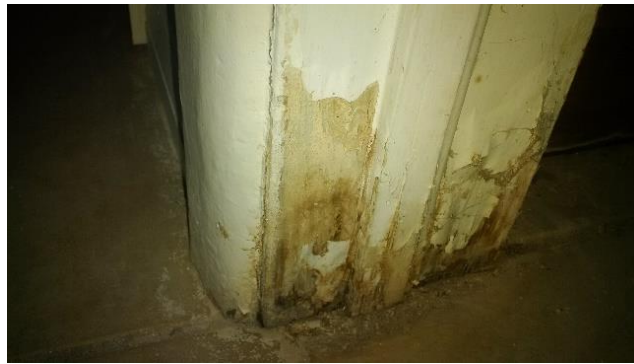
Cracks in a patched wall allowed water to seep into this mobile home
