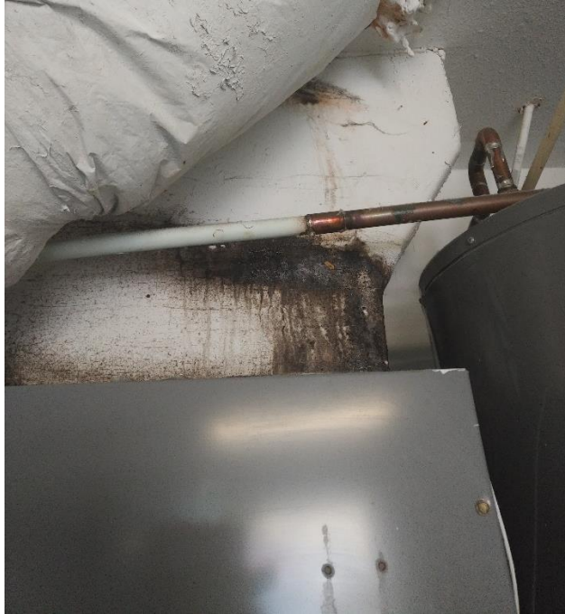
A water leak in an A/C ran down the wall & pipes
